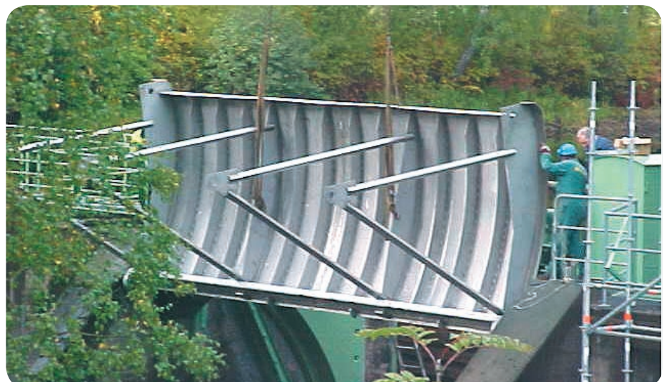
Fig. 5 Stationary structure – floodgate manufactured in LDX 2101 during installation. (Courtesy of Stålmonteringar AB STÅLAB).
