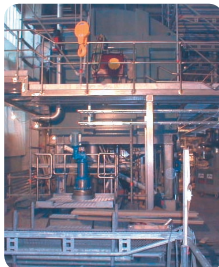
Fig. 3 Stationary steel structure – maintenance platform with hollow sections of austenitic stainless steels (Courtesy of Stålmontering AB STÅLAB).
