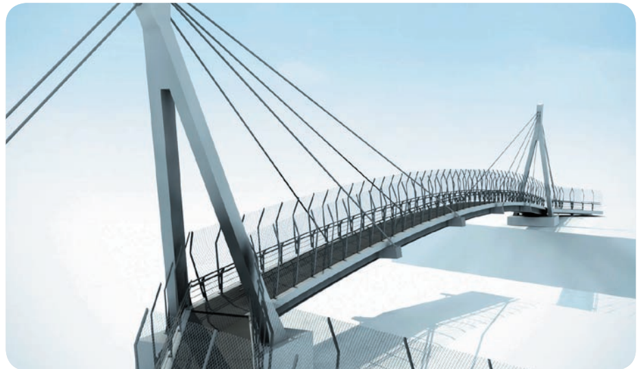
Fig. 4 Stationary steel structure – footbridge to be manufactured in LDX 2101, Ruffolo Bridge, Siena Italy. (Courtesy of SETCO).
