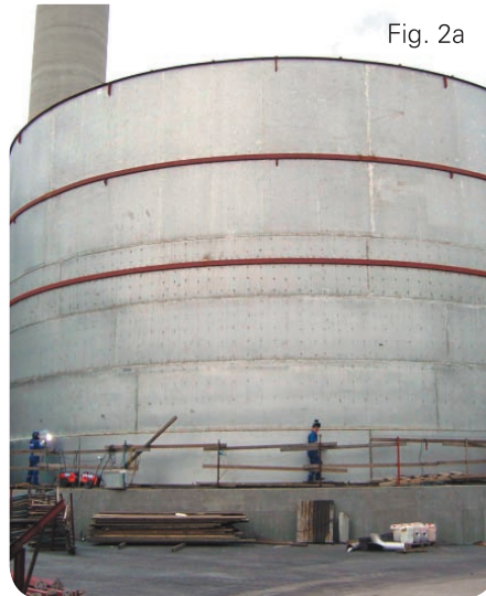
Fig. 2 Process equipment – storage tanks and pressure vessels. The pictures show a white liquor tank in LDX 2101 (Courtesy of YIT), left and the world's largest continuous digester in duplex 2205 (Courtesy of Kvaerner Pulping), right.
